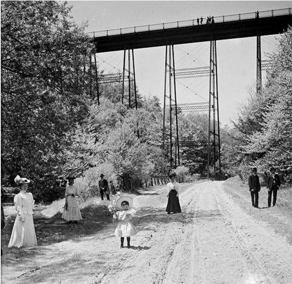
Strollers in the Avoca Ravine beneath the bridge from St. Clair Avenue East to Moore Park, 1911 (City of Toronto Archives)
